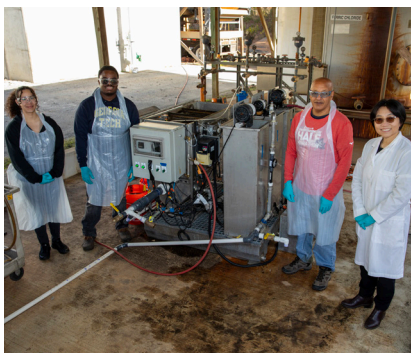
The GTRI team pictured at the Woodstock wastewater treatment plant next to the dissolved air flotation unit it used to test its nanoparticle technology during a recent pilot test.
