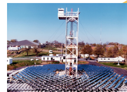
The Advanced Components Test Facility was a 325 kW solar thermal furnace operated by EES for the U.S. Department of Energy.
