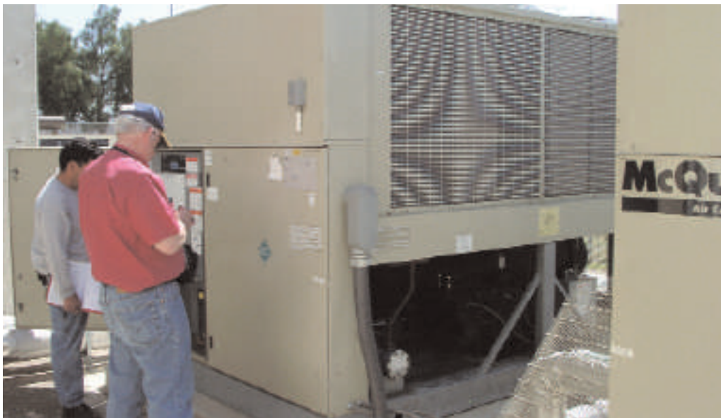
Georgia Tech researchers check an air conditioning unit at the Marine Corps Air Station Miramar in California.
